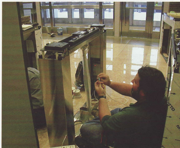
An M.C. Dean, Inc. technician installs the turnstile at USSS.
